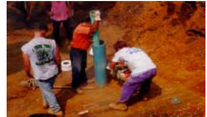
Cutting pipe to lateral elevation
