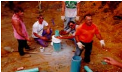
Installing casing cap
