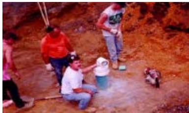
Riser bend in place
