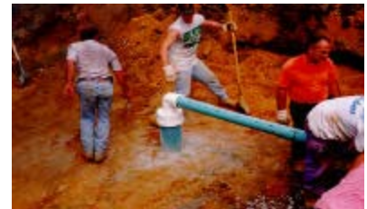
Lateral piping installed
