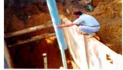
Installing Casing Pipe
