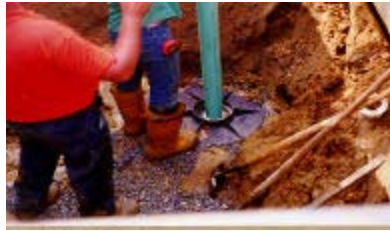
Setting casing shoe & riser
