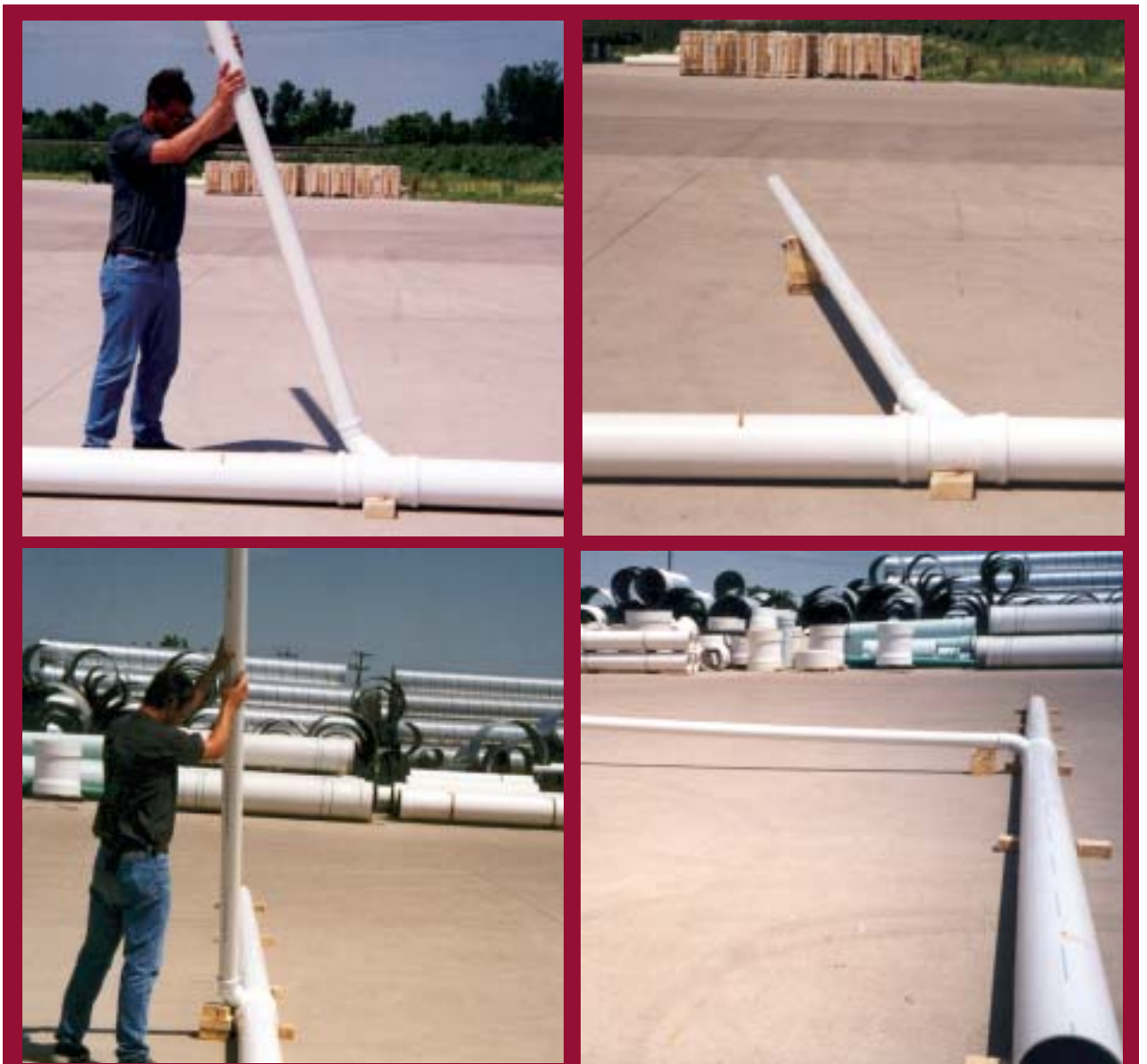
Figure 2 These photographs show a lateral installed with a 45° bend and a wye as sketched in Figure 1.
